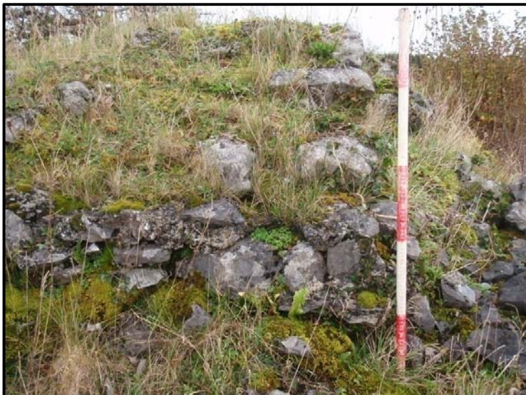
Plate No. 11.4 South-west corner of Moneyduff Castle, showing mortared rubble.
